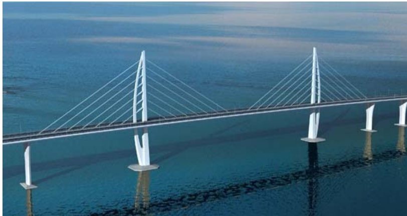
Fig. 2 Jiuzhou Channel Bridge
